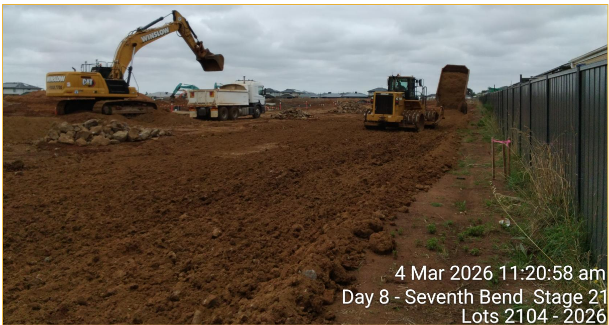
Figure 5: Fill Compaction on Stage 21 (Source: CTGM)
