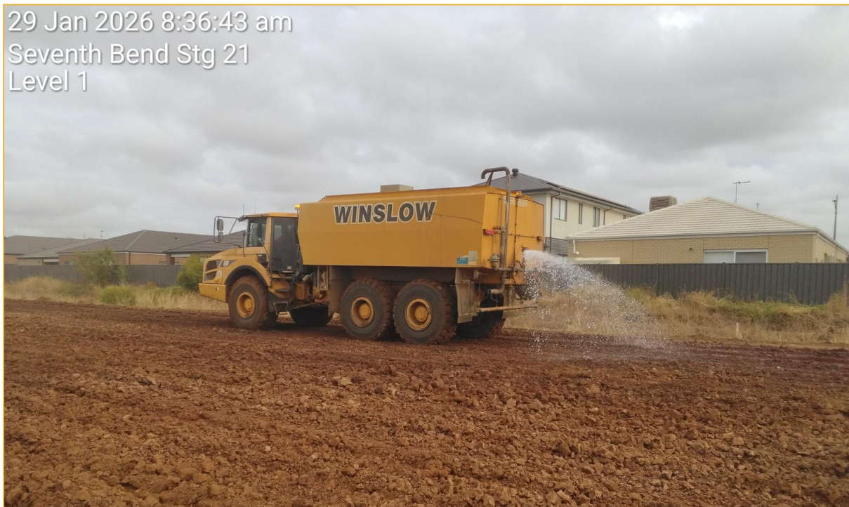
Figure 1: Subgrade Moisture Conditioning Within Stage 21 (Source: CTGM)
