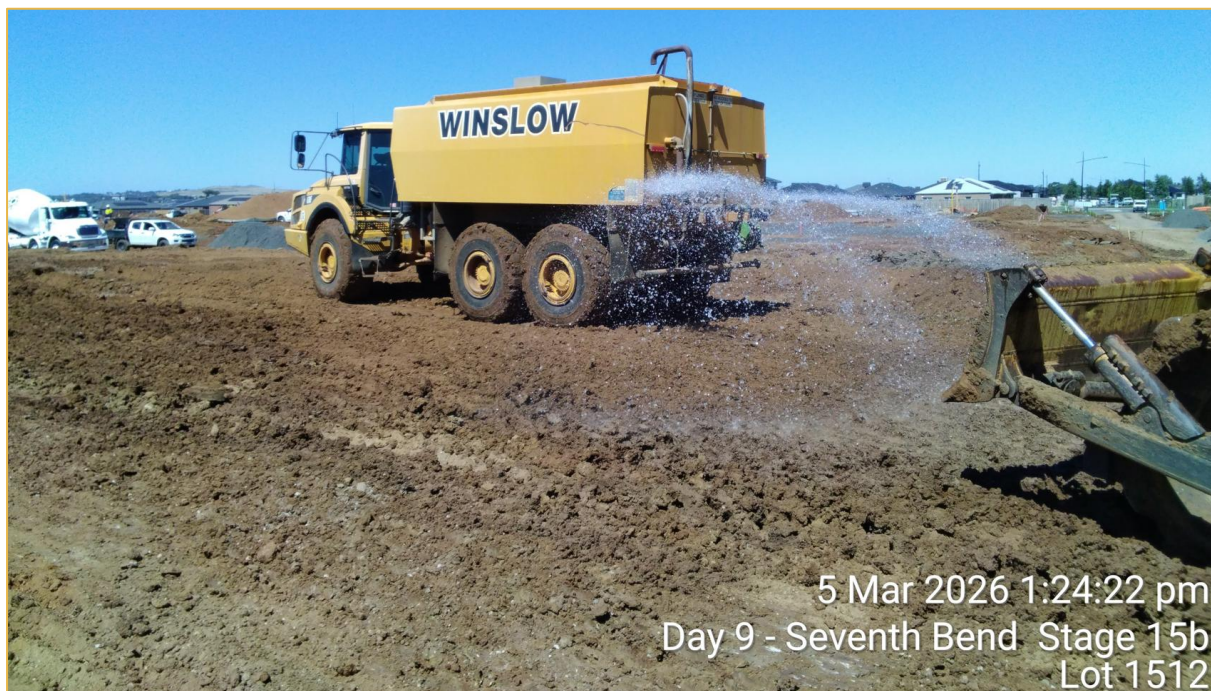
Figure 3: Moisture Conditioning of Fill Material on Stage 15B (Source: CTGM)
