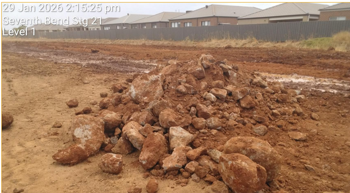
Figure 2: Oversize Particles Removed During Subgrade Preparation (Source: CTGM)
