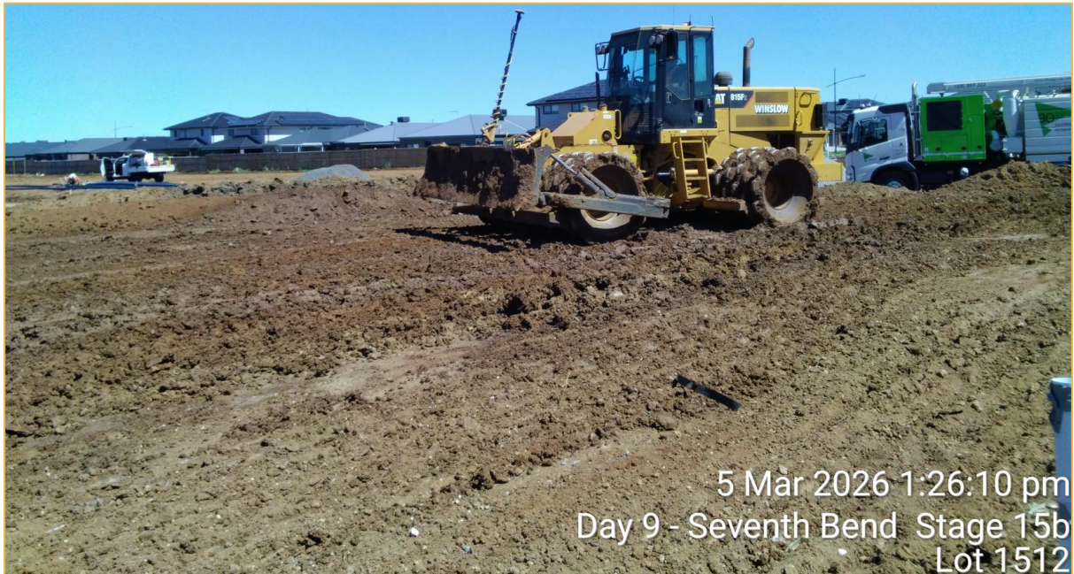
Figure 4: Fill Compaction on Stage 15B (Source: CTGM)
